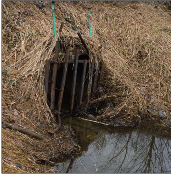
Photo 19: West Sq'ewlets Slough. Facing South with view of culvert that runs under the dike to the Fraser River. Photo taken October 28, 2016.
