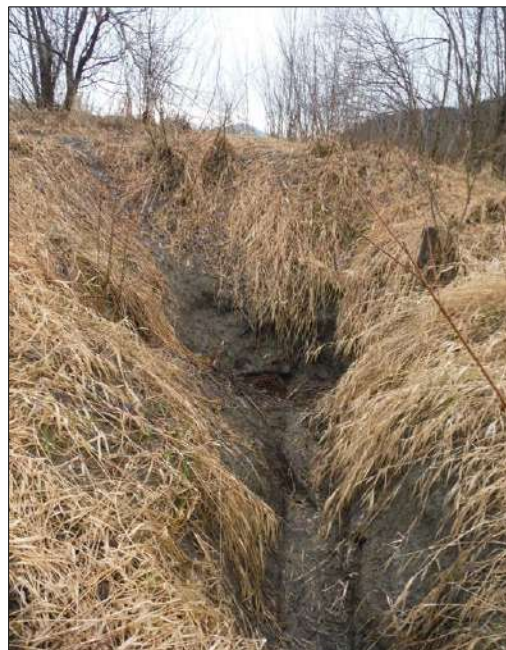
Photo 4: East Sq'ewlets Slough. Facing South with a view of the de-watered, entrenched channel leading to a culvert with mesh screen that runs under a dike to the Fraser River. Photo taken October 27, 2016.
