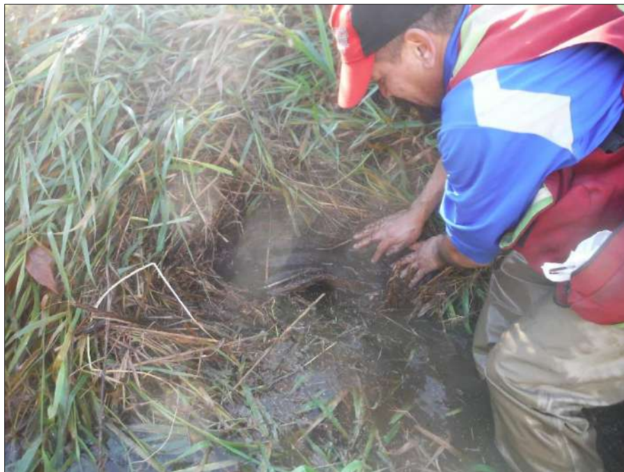
Photo 2: Bateson Slough North. Facing South with view of culvert that connects to Bateson Slough South under Lougheed Highway. Photo taken October 27, 2016.
