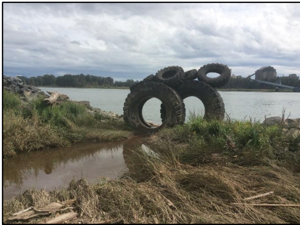
Image 3: Tire log debris protection structure. Compensation site 10-002-A. July 28th, 2015
