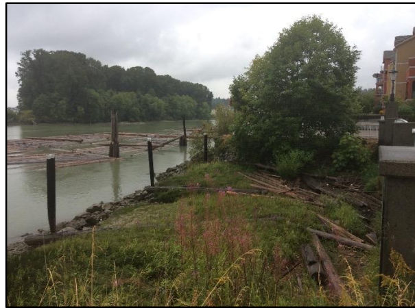
Image 4: Posts as log debris protection. Compensation site 01-003-B. July 24th, 2015
