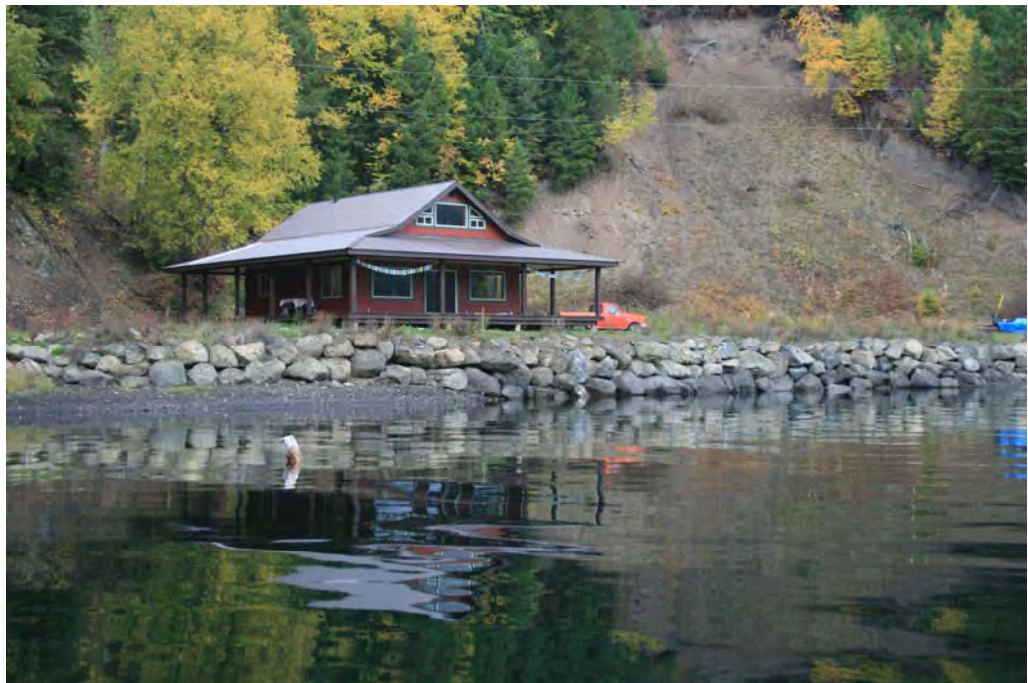
Photo 1: Looking towards a retaining wall and associated anthropogenic impacts.
