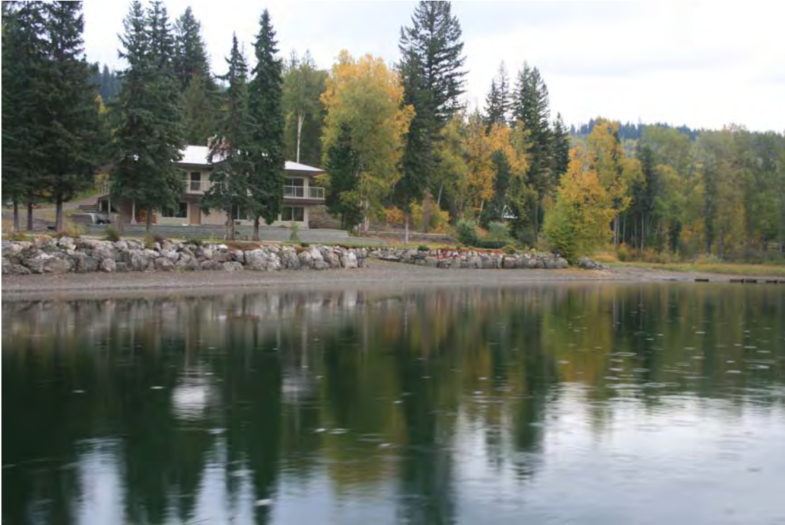
Photo 7: Looking towards an example of a retaining wall and associated anthropogenic impacts occurring along the West Arm of Quesnel Lake.
