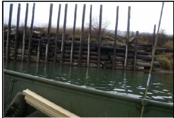
Rip rap and Bank Stabilization
