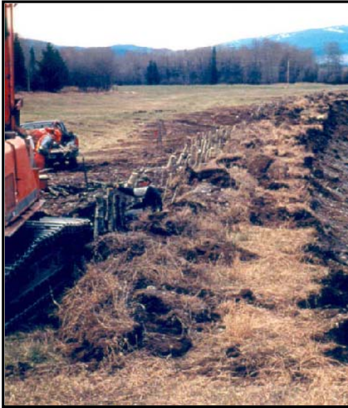
Live palisade using cottonwood to restore mid flood bench riparian ecosystems and to promote bank stability (Photos by D. Polster).
