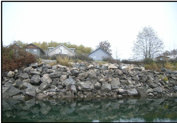
Rip rap and Bank Stabilization
