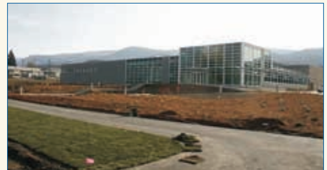
new state-of-the-art River Street Water treatment Plant in Kamloops.
