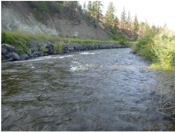
Rip rap and Bank Stabilization
