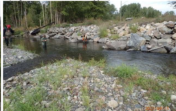
Rip rap and Bank Stabilization
