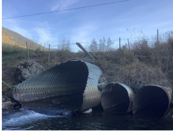
Priority Restoration Site (i.e., culverts barrier to fish passage)
