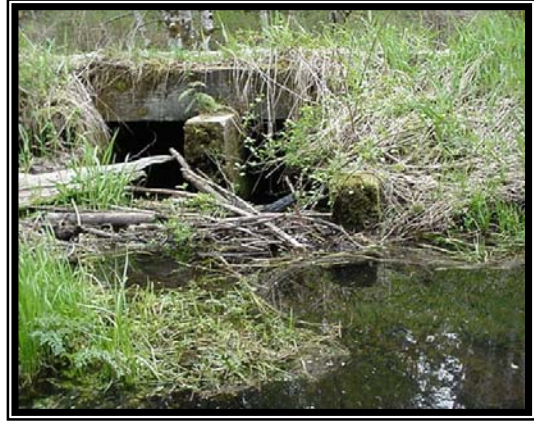
Figure 9. Downstream at Culvert of Reach 1, Segment 1
