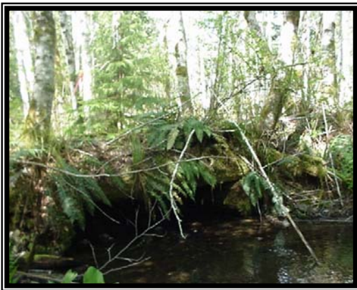
Figure 5. Box Culvert in Reach 2, Segment 2
